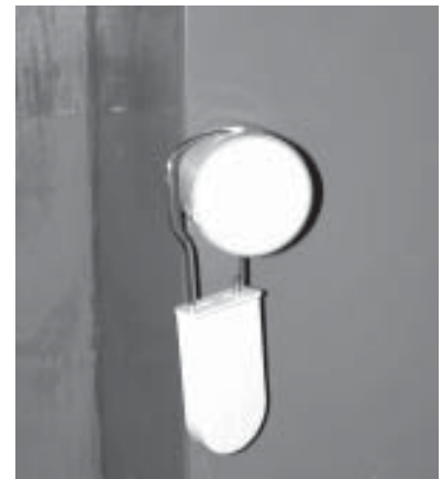
Step 3 - Sleeve larger cap over small cap and insert meter seal.
