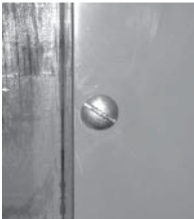
Step 1 - Remove existing panel screw.
