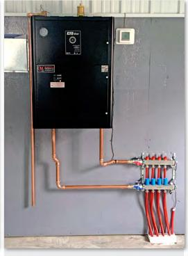
The EZBoiler® series is a clean and simple installation each and every time.
